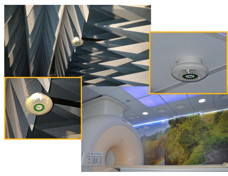
The OAS-S is an optical alarm system for smoke detection, to be mounted in an anechoic chamber or in proximity of the toroid of the magnetic resonance imaging. The OAS will eventually report the alarm through a light signal. Thanks to its external fiber optic connection and its battery supply, the OAS-S has no emissions of any kind so both the resonance artifact and the anechoic chamber measurement are not affected.
